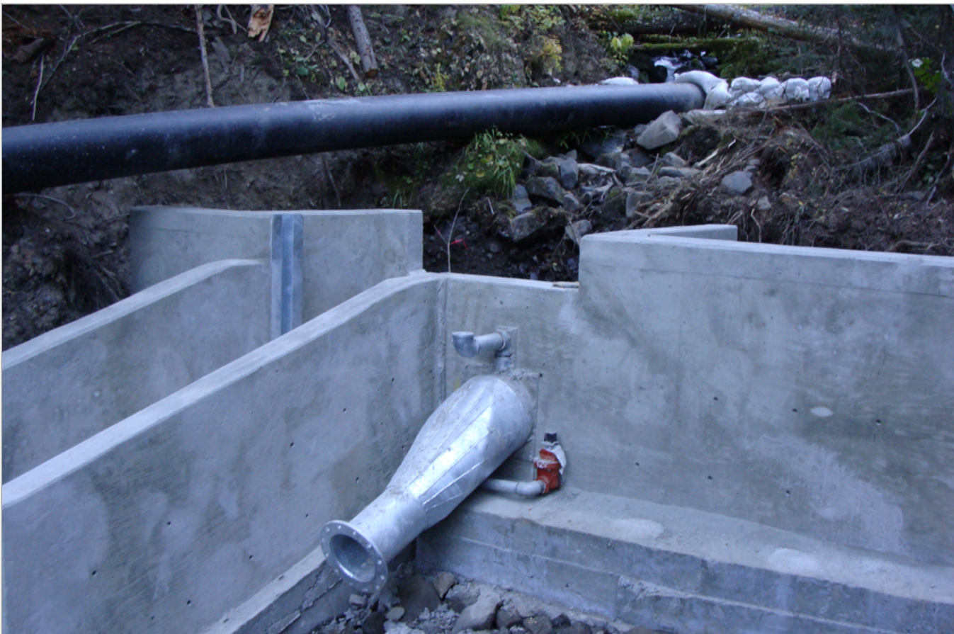
Photo of Lake Creek dam during construction. The fish passage channel is on the left side of the photo.
